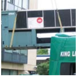
The old chiller is removed from the building
