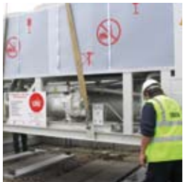
Final positioning of the new chiller takes place
